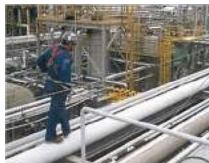
Before a fall-arrest system is used, the work area should be inspected to ensure there are no obstructions in the potential fall path.
